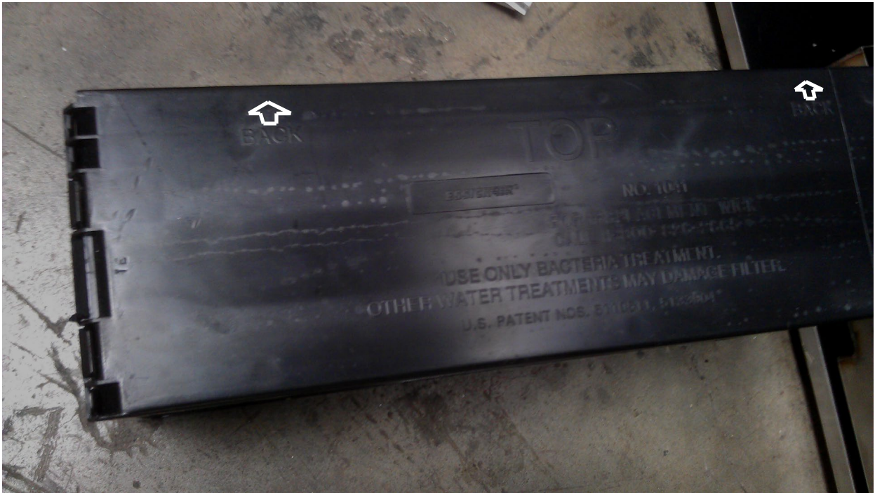
Figure 6 - Wick orientation. Arrows denote the side that should be facing the condensing unit.
